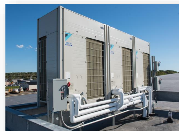
Presque Isle Community Building
